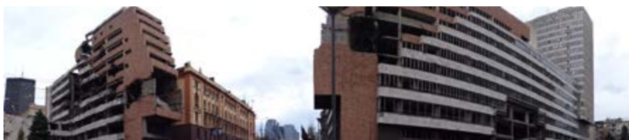
Figure 2.58. Panoramic view of the damage caused to Dobrović's Federal Ministry of Defense buildings by NATO bombing. These were the strongest signature of socialist urbanism in the tissue of old Belgrade. Left standing as a reminder of the bombing, they were finally demolished in 2015. Photo credit: Adam Jones (Creative Commons Attribution-Share Alike 2.0 Generic license - https://commons.wikimedia.org/wiki/File:Panorama_of_Buildings_Damaged_in_1999_Kosovo_War_-_Belgrade_-_Serbia_(15803615912).jpg )
