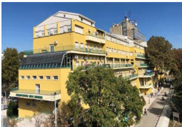
Figure 2.53. Altered form of the Children's Hospital on Tiršova Street. Photo credit: Milan Zloković (via the Milan Zloković Foundation).
