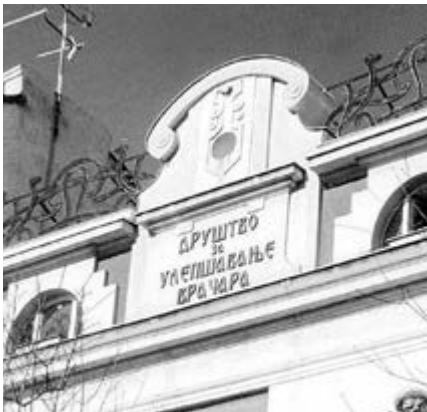
Figure 2.105. Building of the Society for the Embellishment of Vračar on Njegoševa Street. The “Miroslav” typeface is more convincing on older buildings. Photo credit: author.
