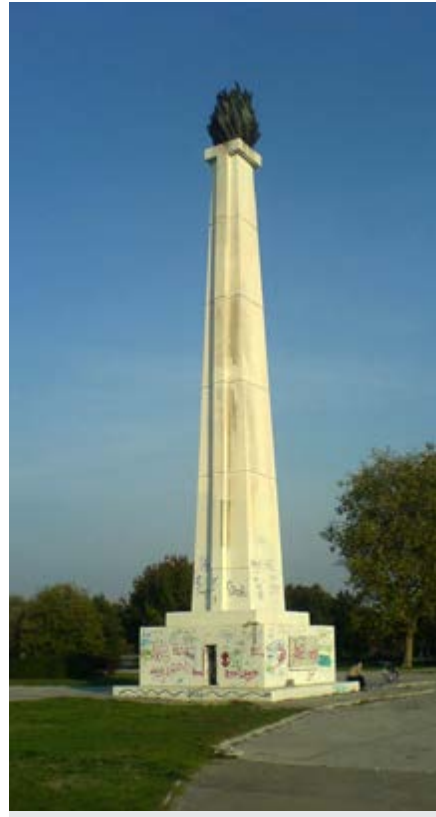
Figure 2.146. After Milošević was removed from office, the “Obelisk of the Eternal Flame” started accumulating graffiti on its base and brass letters from the inscription were stolen, making the text unreadable. Because the Obelisk had been built without a legal permit, it was not protected by the Institute for the Protection of Cultural Monuments. This was sorted out years later and the monument was finally cleaned and repaired in 2019. Photo credit: Pinki (Serbian Wikipedia), released into the public domain.
