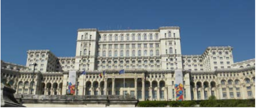
Figure 2.140. Ceaușescu's People's Palace in Bucharest: the biggest building in Europe and second-biggest in the world. This is only the apex of the project which included the long Victory of Socialism Boulevard with large multifunction buildings, coordinated in design, lining both sides of the street. Photo credit: Vi Ko (CC BY-SA 4.0).
